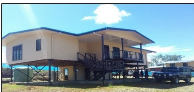
Judge House completed and awaiting service connections and furniture
