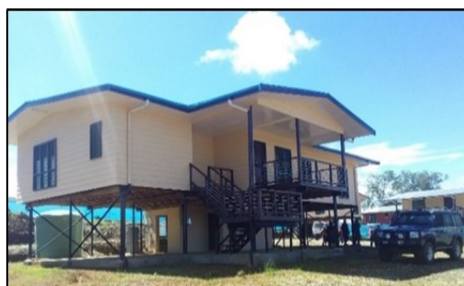
One of the four houses completed by contractor 1
